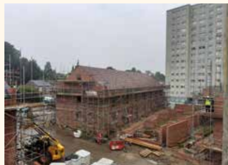
Progress on site
